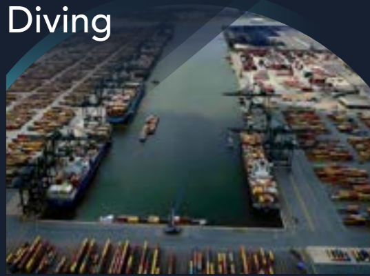
Project: Covestro Antwerp - Splash zone conservation jetty piles
