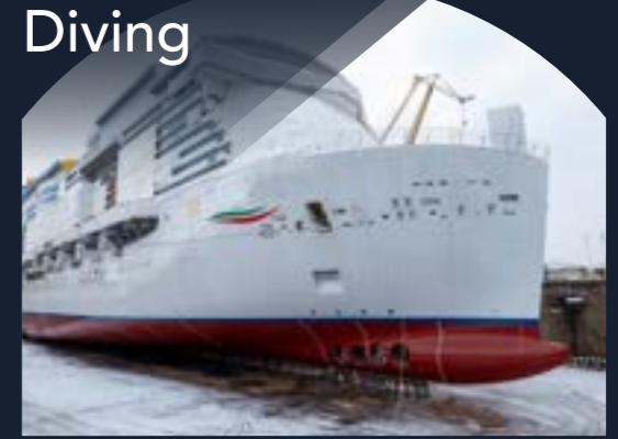
Project: Cruise vessel - Emergency repair after grounding
