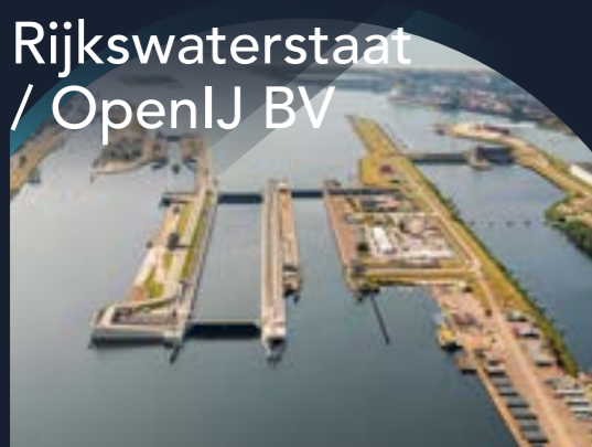
Project: Zeesluifs IJmuiden - Conservation sheet piles
