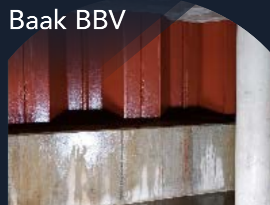
Project: Holland Tunnel - Water cellar conservation sheet piles
