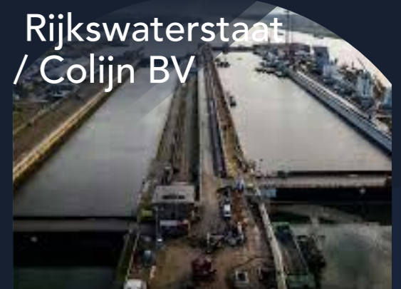
Project: Selective extraction at sea lock IJmuiden - conservation waterline sheetpiles
