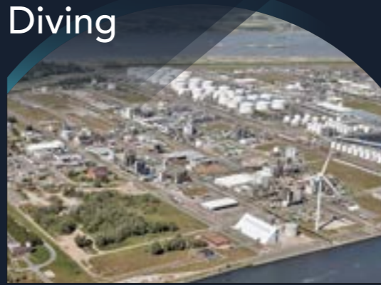
Project: Evonik Antwerp - FiFi tank internal refit
